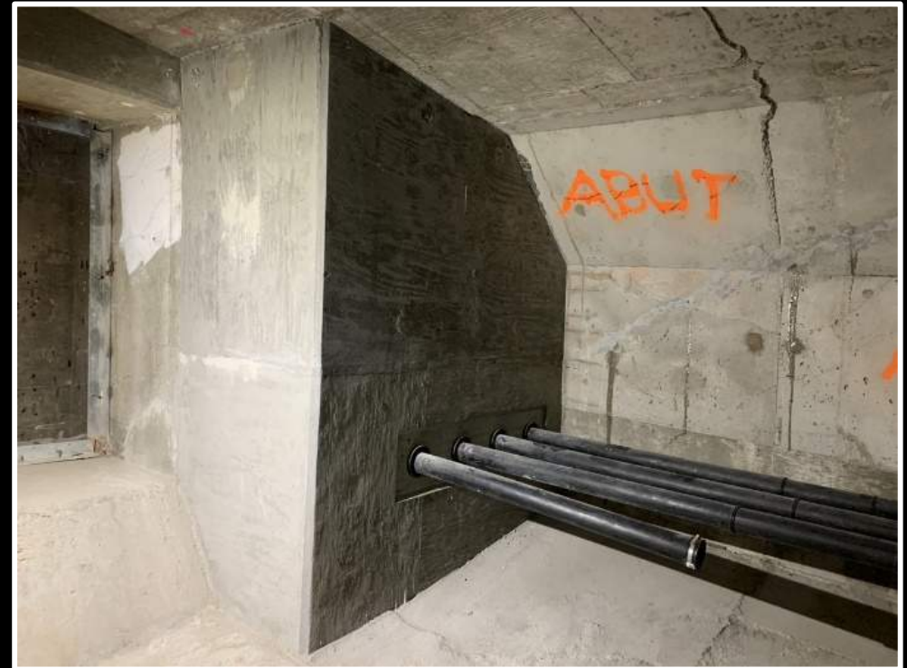
Completed Diaphragm Extension
