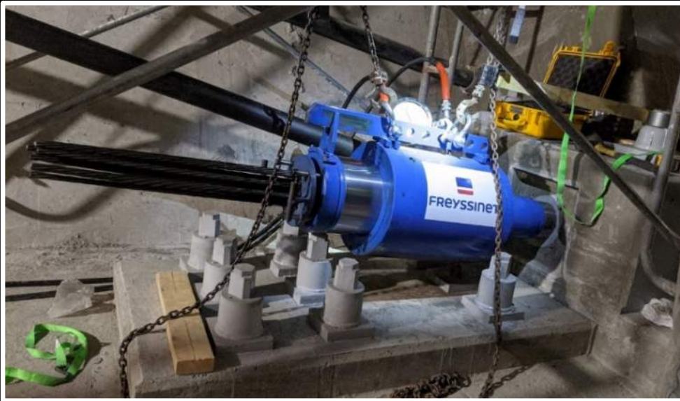
Span 16 Stressing – Fit like a glove
