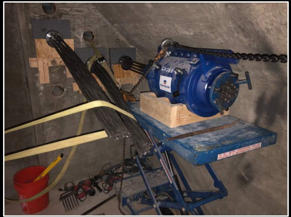
Tendon Stressing at Pier 1 Diaphragm
