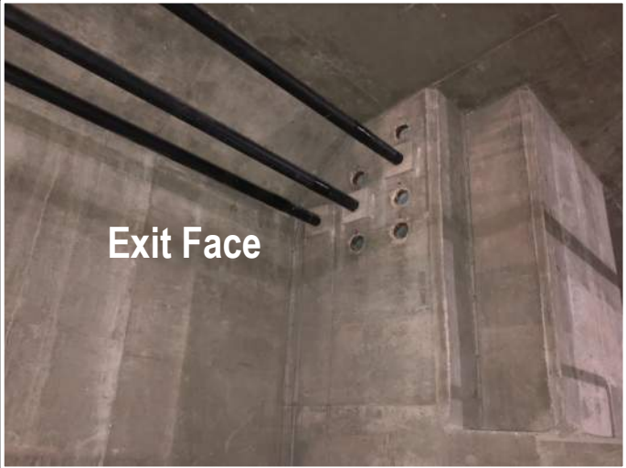
Anchor Face, Pier 1 Diaphragm
