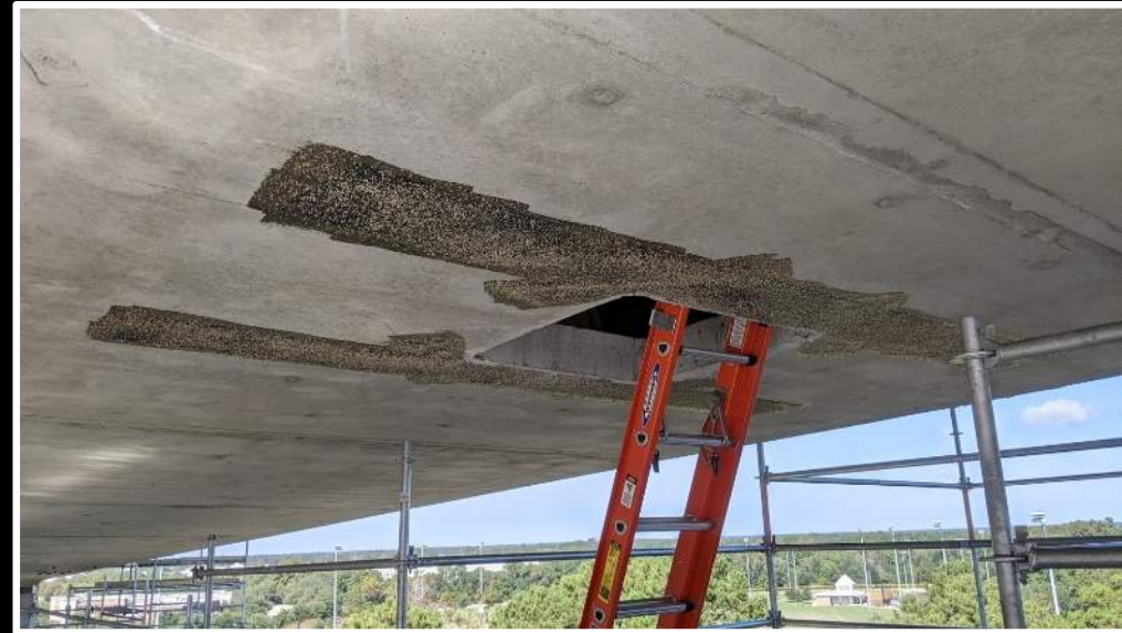
CFRP reinforcing at new access opening
