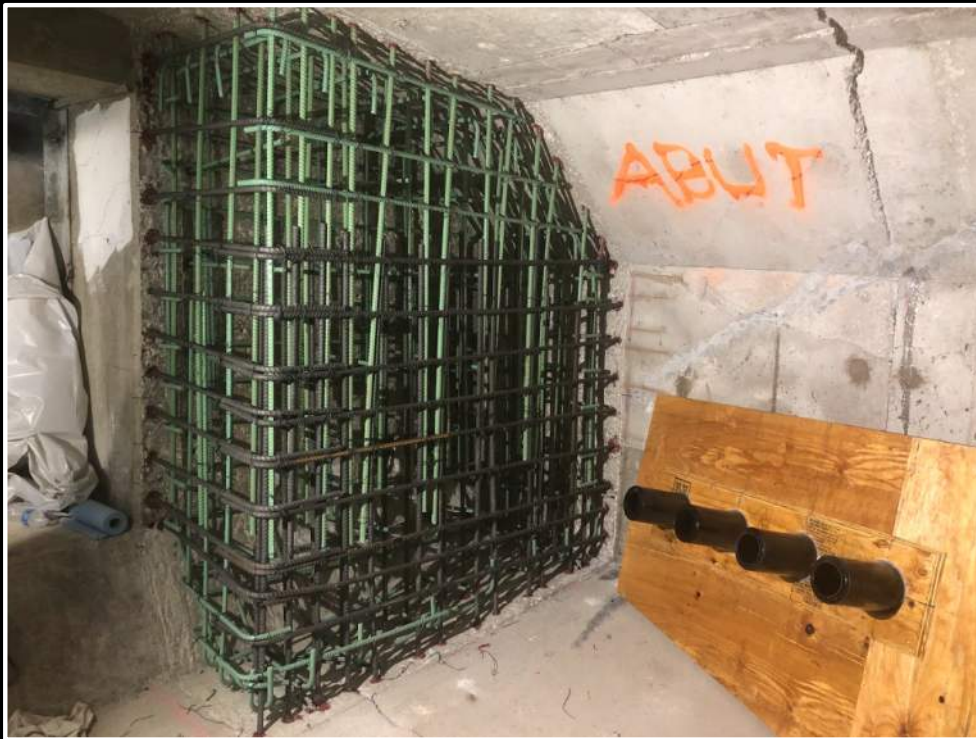
Diaphragm Extension – Rebar Cage
